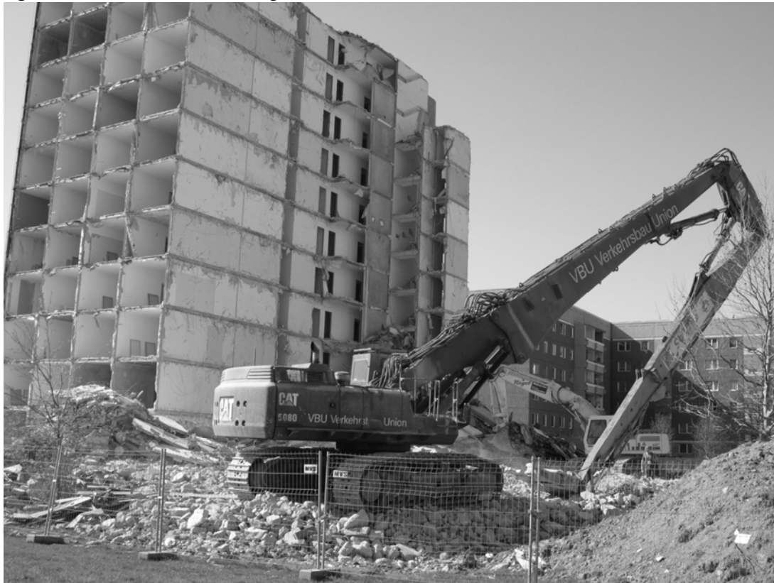
Figure 3.4.7: Demolition of Housing
