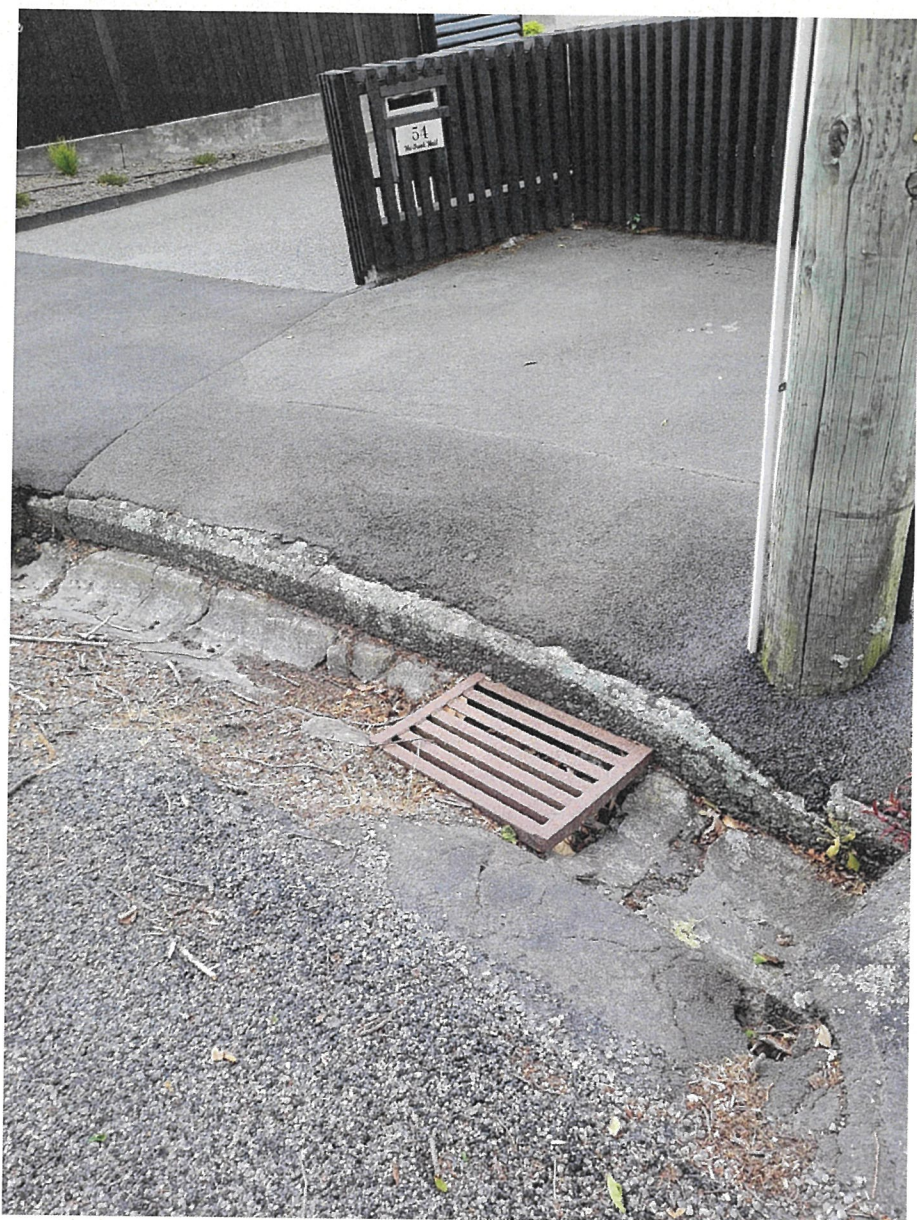
Wairarapa Terrace – road gutter discharge to the creek between 52 & 54.
