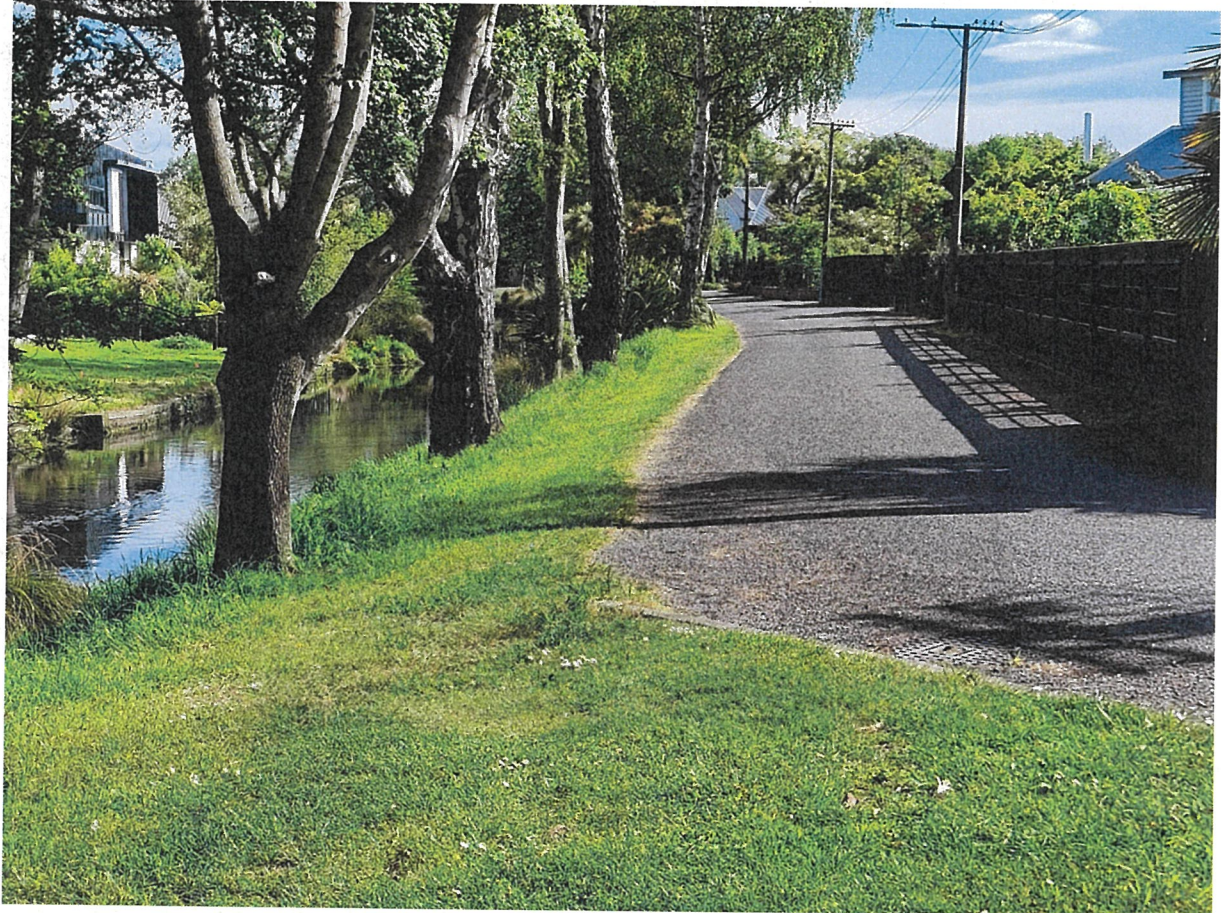
Photo 8 Wairarapa Terrace higher bank – narrowing the flood plain on the low bank raises water levels .
