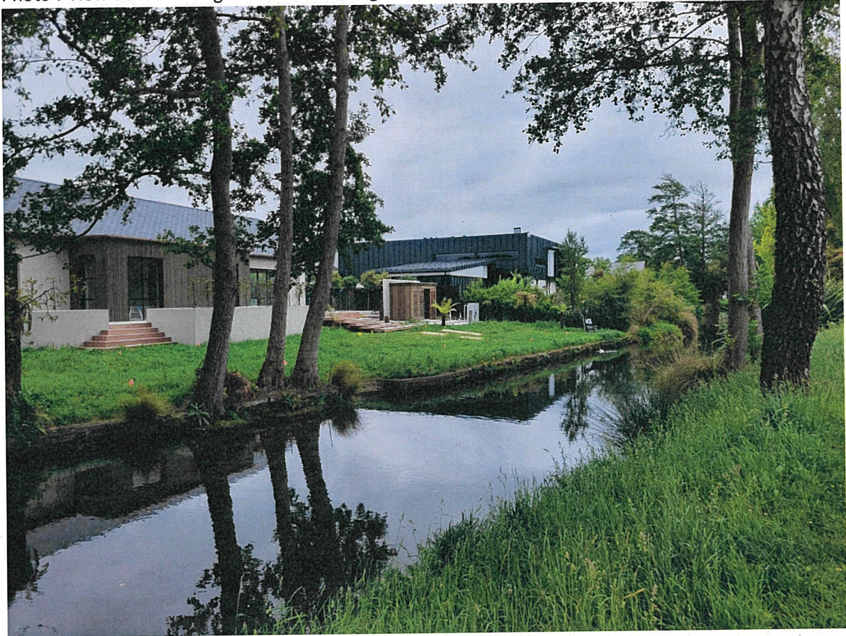
Photo 7 New Builds are higher and the raising of the slope narrows the stream flood area.
