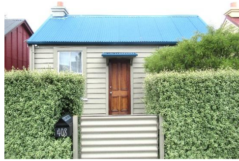
408 Montreal St: renovated cottage on 122m 2
