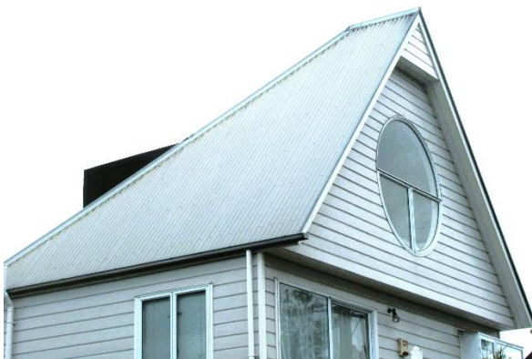
Use of exaggerated recession plane to allow 3-storey townhouse on an infill section of 148m 2 (49A Gracefield Avenue)
