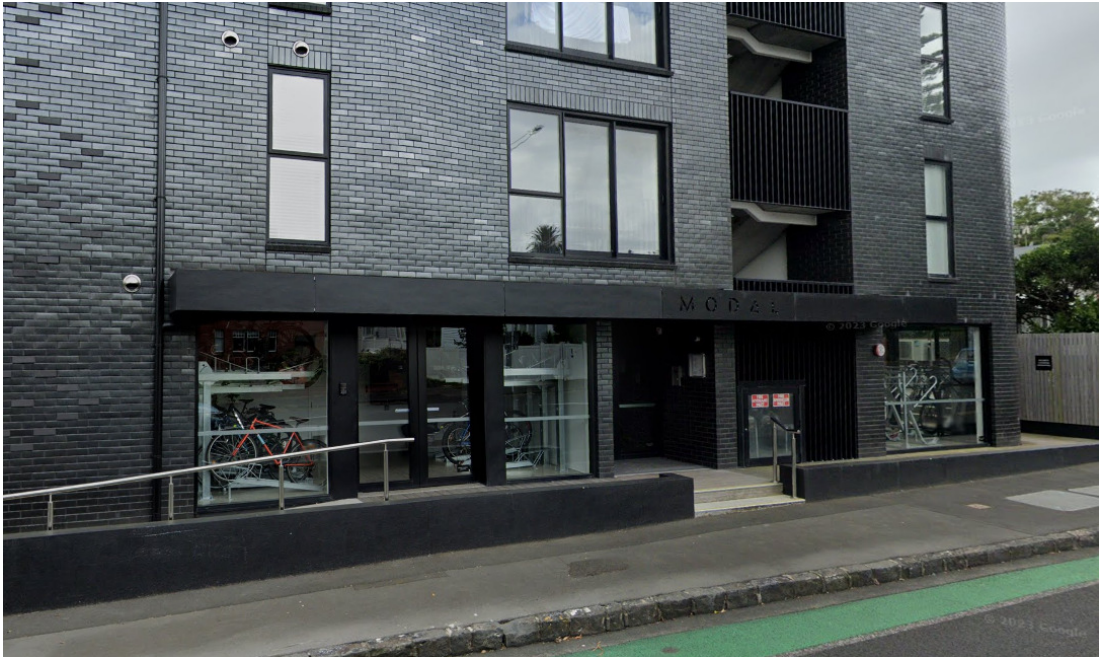
Figure 1: Residential development with integrated, at grade bike storage visible on the ground floor 26
