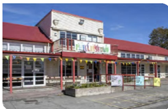
Phillipstown Community Hub
