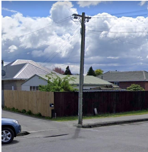
Garage built under the overhead service main.
