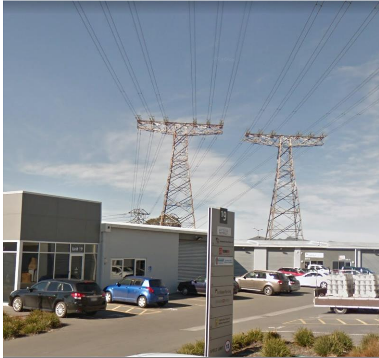
Tower lines – built up area – 66,000V
