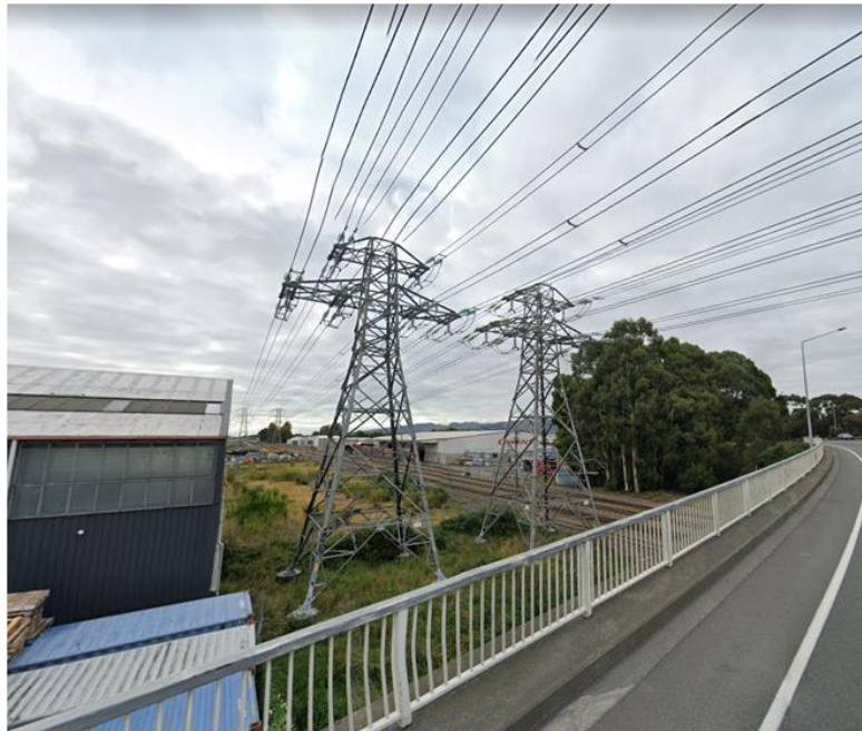
Tower lines – built up area – 66,000V
