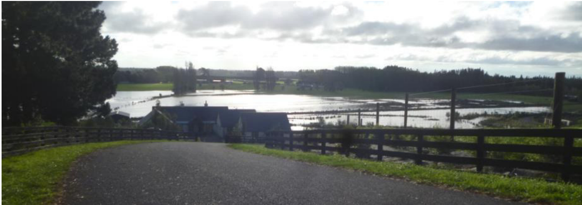
Stackwoods drain area, 30 April 2014
