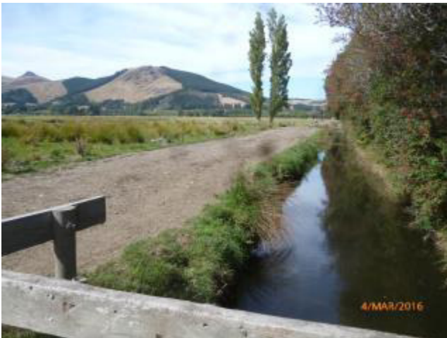
Stackwoods Drain near Woods Drain. Water levels flat. Land to left of picture only marginally above water level
