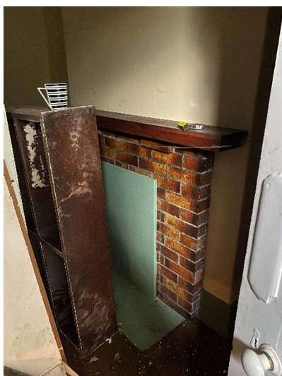
Fireplace that replaced one of the original
