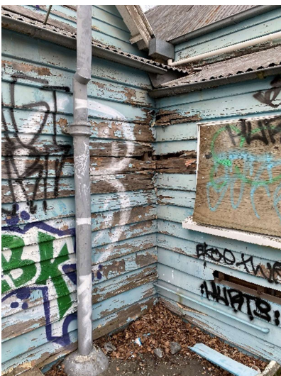
Cladding deterioration
