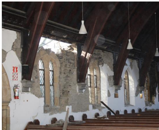
Fig 5. Church Nave (South side) - Internal View - .
