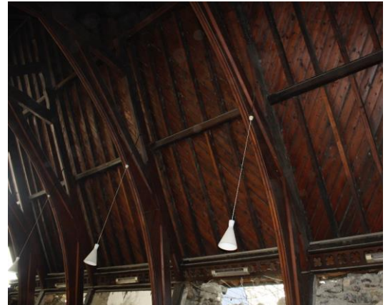
Fig 2. Church Roof Structure - Internal View-.
