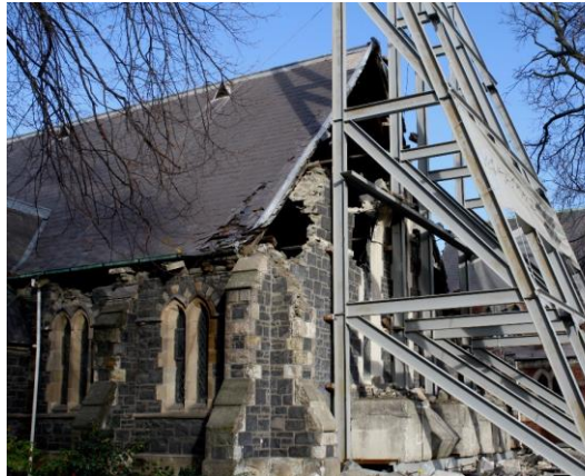
Fig 1. West gable end - External View - .
