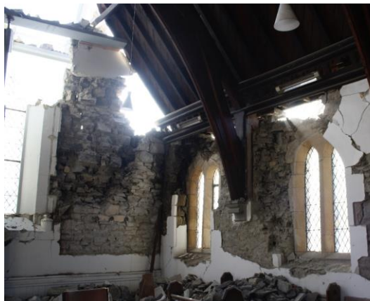
Fig 3. Church North- West Corner - Internal View - .
