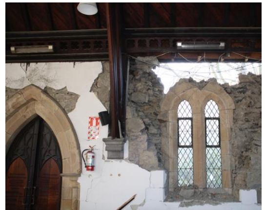
Fig 6. Church Nave (South side) - Internal View - .
