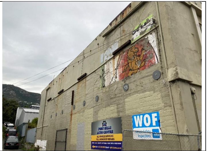
Photo 2 – View from West side wall
