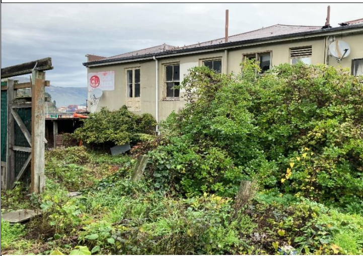
Photo 5–View from Rear Side (North)
