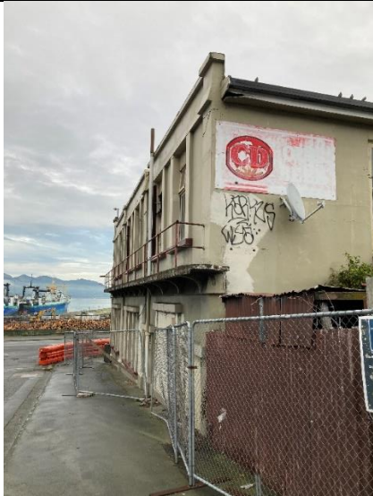
Photo 3 – View from East side wall
