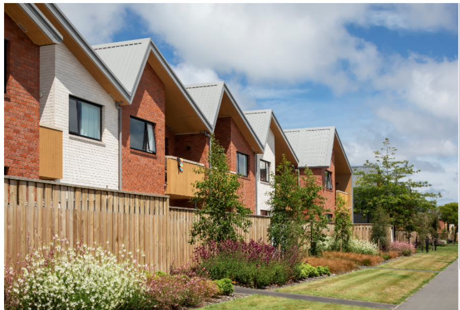
Figure 2. OCHT social housing development - Brougham Street
