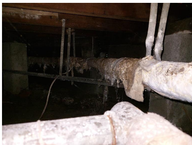
Photo 3: Subfloor – Lagged pipes
