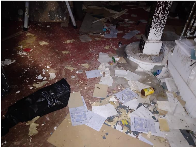
Photo 15: Evidence of condition – Ground Floor Lobby
