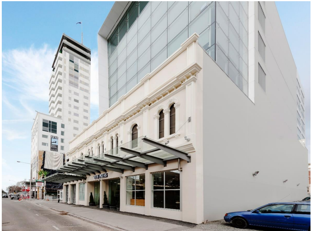
Photograph 6: 158 Gloucester Street, Christchurch
