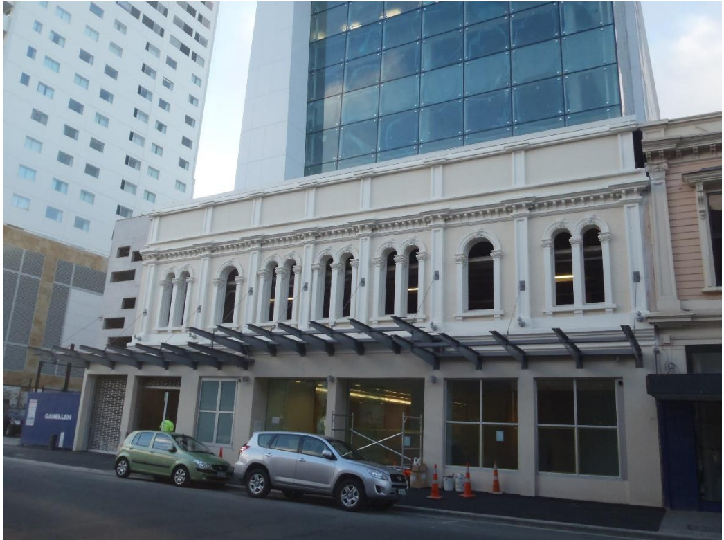
Photograph 1: 158 Gloucester Street, Christchurch – pre February earthquake
