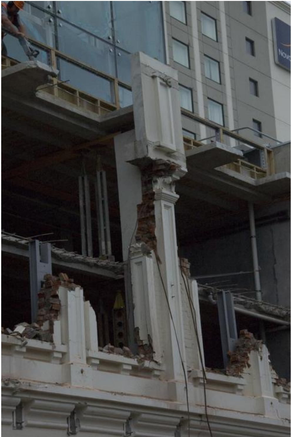
Photograph 4: 158 Gloucester Street, Christchurch – during demolition
