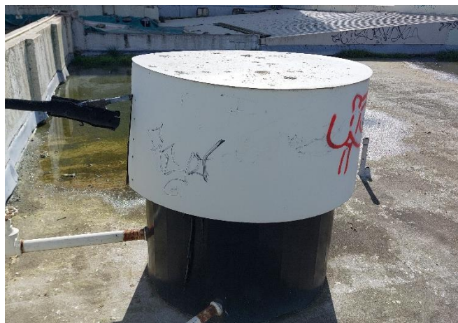
Photo 20: Evidence of condition – Water tank
