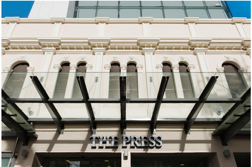
Photograph 5: 158 Gloucester Street, Christchurch
