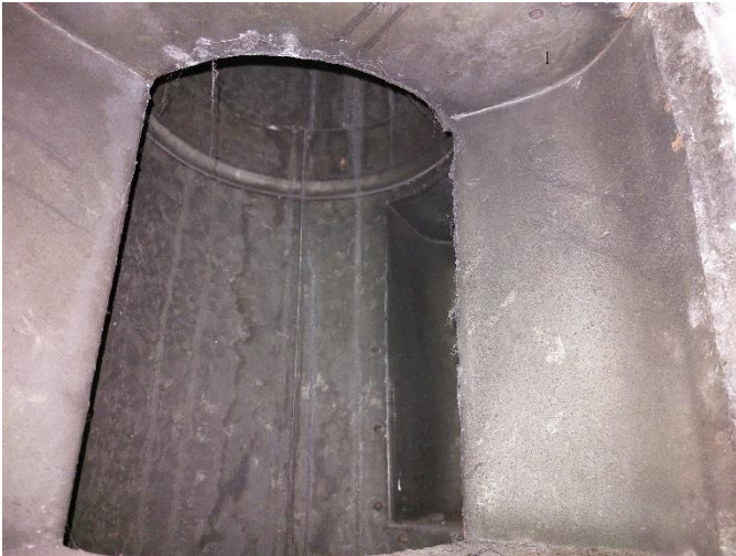
Photo 25: Evidence of condition - Flue within wall in Room 21
