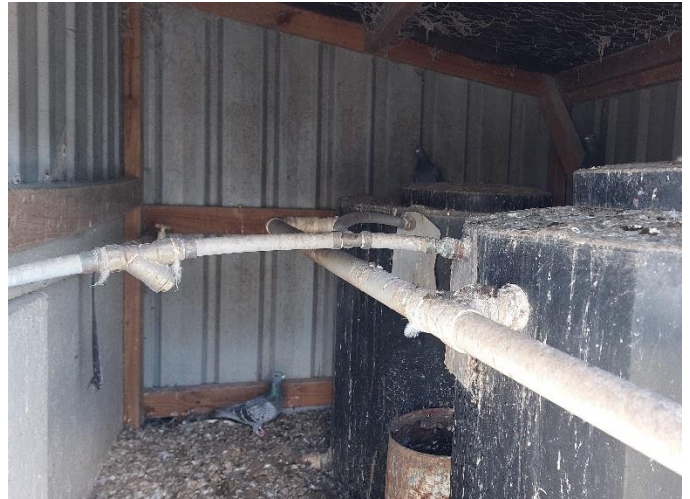
Photo 26: Evidence of condition - Water tanks on roof
