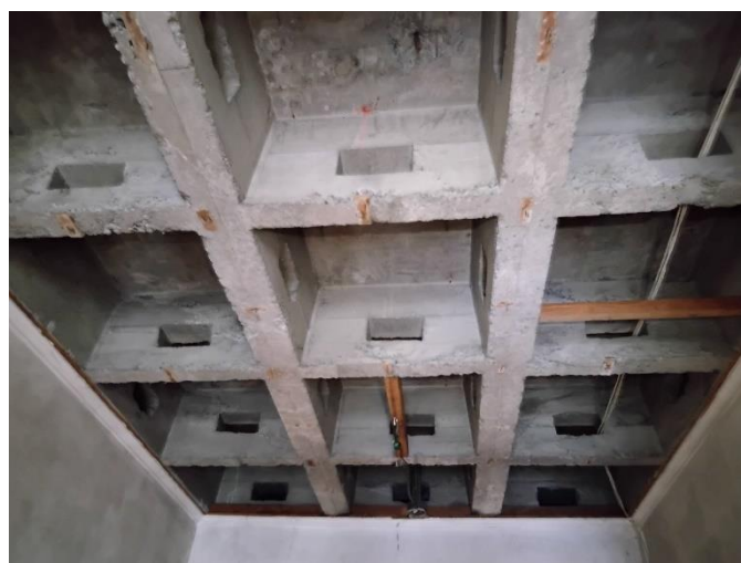
Photo 4: Example of space above ceiling panels
