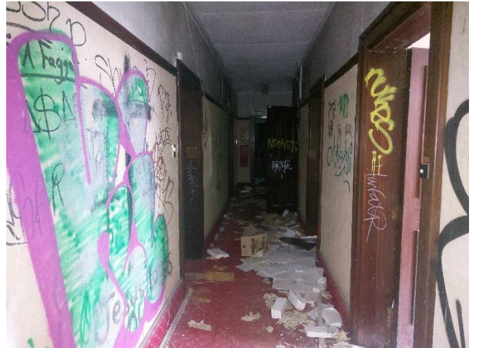
Photo 16: Evidence of condition – First Floor Hallway
