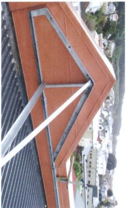
Steel elements added to brace parapets
