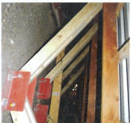
New timber bracing installed inside roof to support parapet bracing
