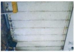
NSM-CFRP strips added to interior partition walls
