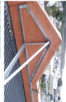
Steel elements added to brace parapets
