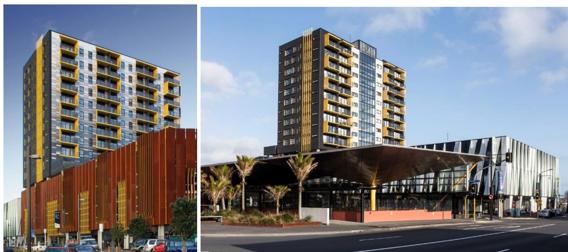
Figure 42 – The transformational-led Merchant Quarter includes approx. 50 metres in height, is located adjacent to the redeveloped and trenched New Lynn Station 44
