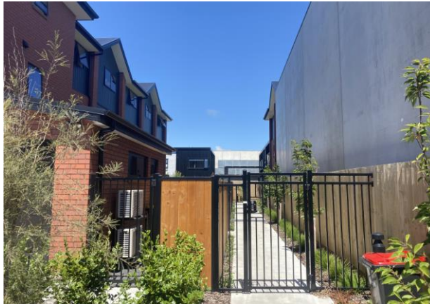
Figure 10 – Photo from Aberdeen Street of the blind corner pedestrian access down to terraces in behind an existing building – citing CPTED issues not currently covered in the CCMUZ. RMA/2021/236
