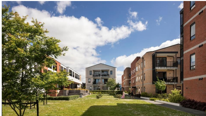
Figure 21 – Bernoulli gardens, whilst only up to 4 storeys provides for the three factors of a high quality living environment.
