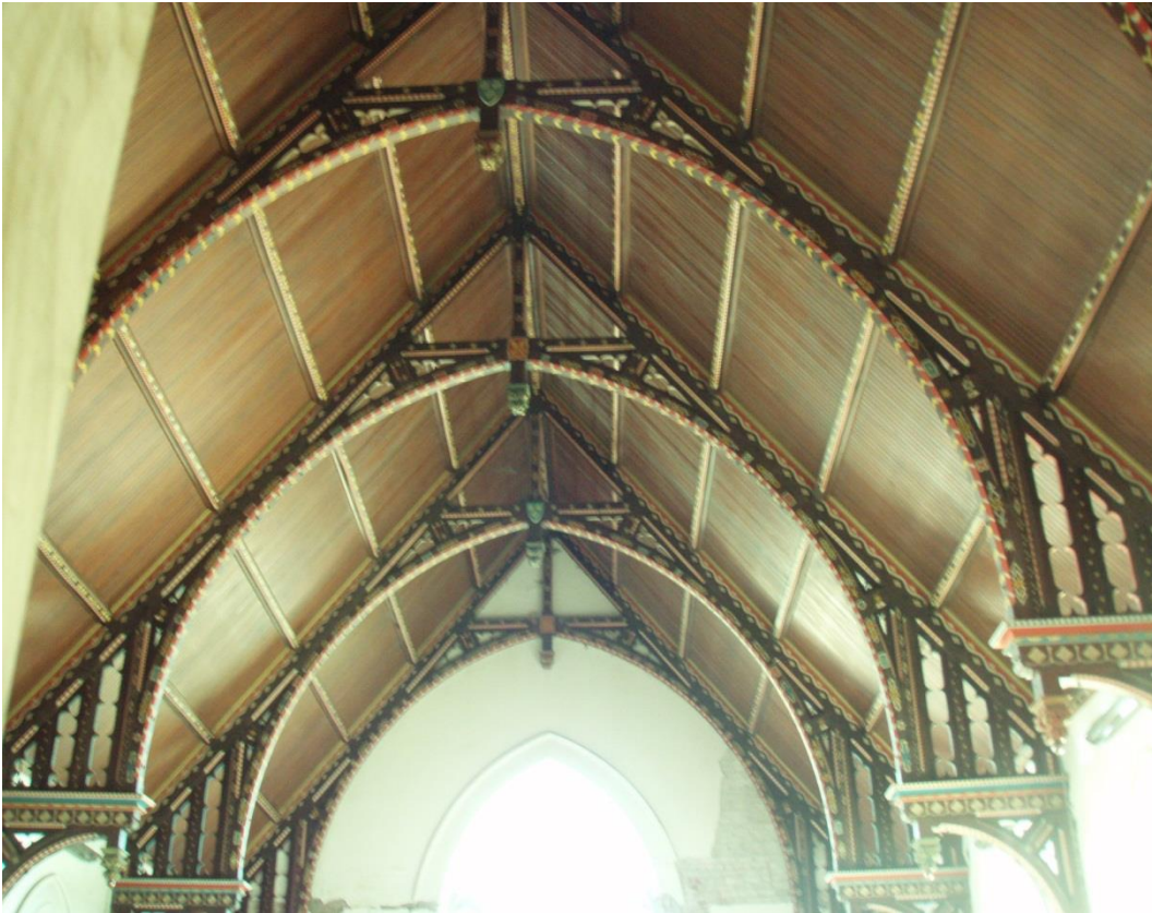
Photo 7 – Interior wood work
