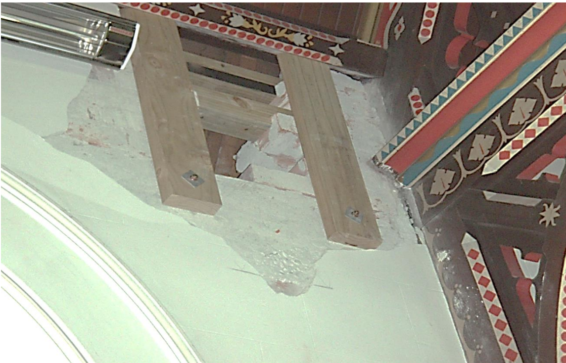
Photo 3a – brick work along top of side walls (opened for investigation purposes)
