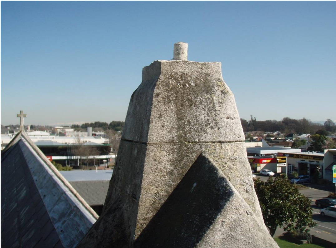
Photo 5b – view at roof level looking from chance arch (cross support will need stitching)
