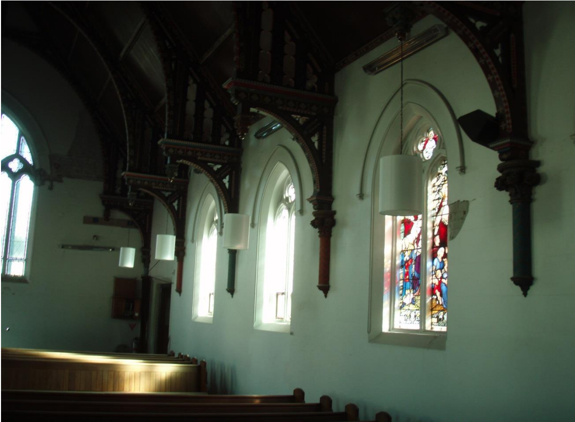
Photo 3 – general view of nave side walls
