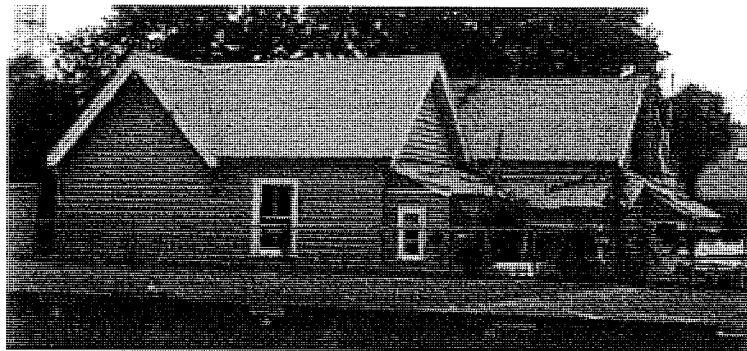
“Cross gable” roof form. Note twin gables at rear.
