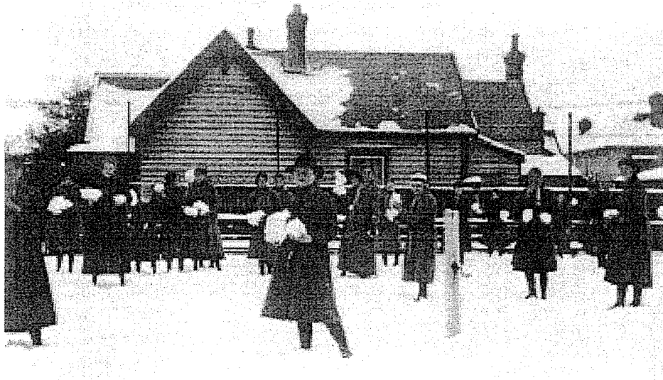
Undated early photograph of the cottage. Note slate roofs, chimneys and bullnose verandah at left of photograph. Note also evidence of earlier colour scheme.
