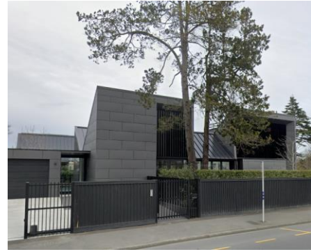
Figure 4: Architectural form and detailing with limited reference to character attributes.
