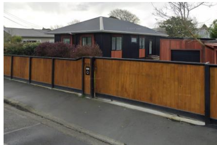
Figure 5: Reclad of exterior contrasts with character.
