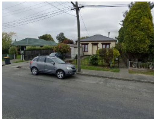
Villa next to 50's properties – Neil Street
