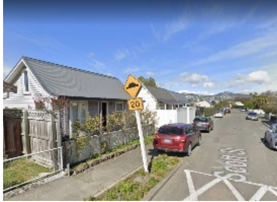
Scott Street workers cottages
