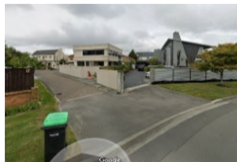
Mixed roof forms Image source: Google Streetview
