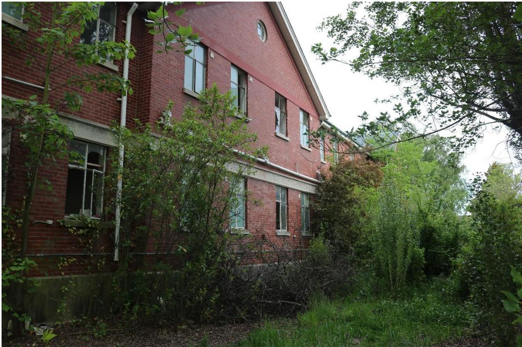
Photo taken 5<sup>th</sup> Nov 2021. Broken windows and unchecked vegetation growth to fence line.
