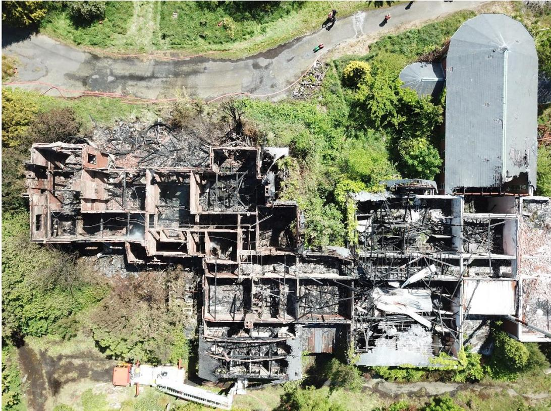
Total loss of all structural floor and roof elements, across ground and first floor areas.
