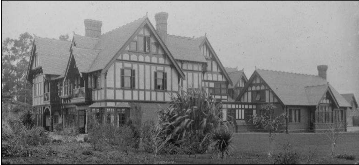
Historical view of Daresbury. Note chimneys.
