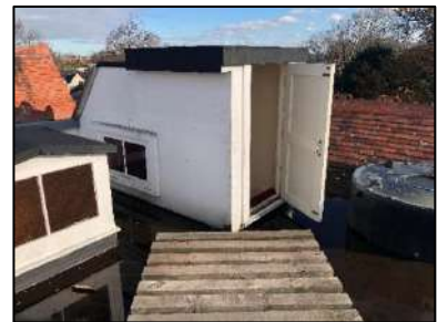
Views of roofscape. Note areas of metal trough roofing and membrane roofing with water ponding. The photograph at right shows the roof access hatch which appears to be original.
