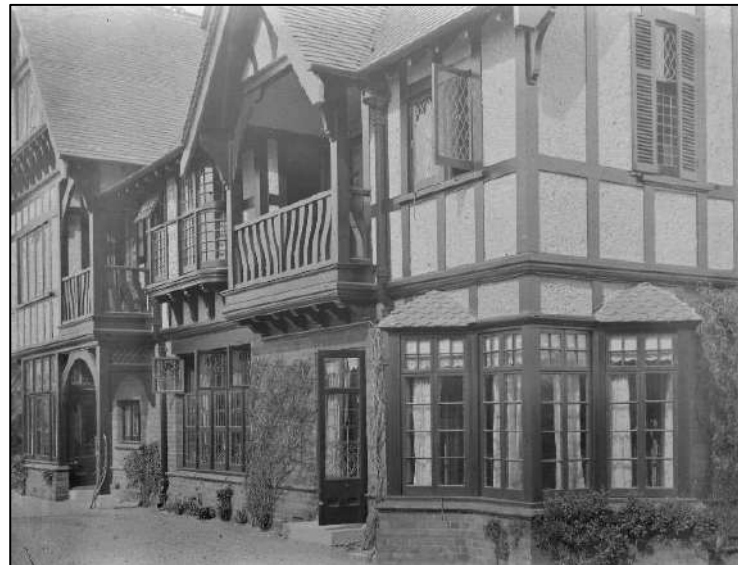
Close up of main entrance (left) and view of north west corner (right). Note corner window in drawing room and balcony in gable end, now infilled with a window.
