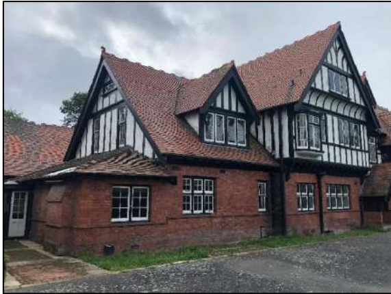
View from north east.
