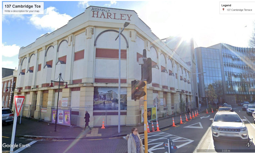
Figure 2 Google Earth photos of building south-east elevation
