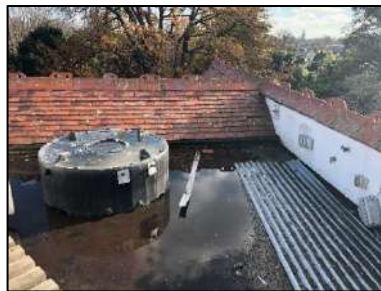
Views of roofscape. Note areas of metal trough roofing and membrane roofing with water ponding. The photograph at right shows the roof access hatch which appears to be original.
