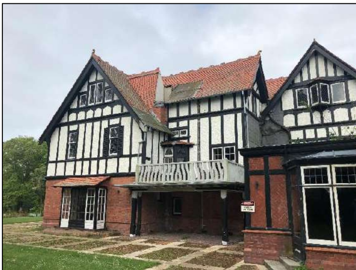
West elevation (left). Note plywood patch on roof indicating former location of chimney.
