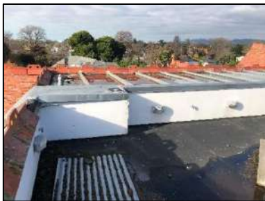
Views of roofscape. Note areas of metal trough roofing and membrane roofing with water ponding. The photograph at right shows the roof access hatch which appears to be original.
