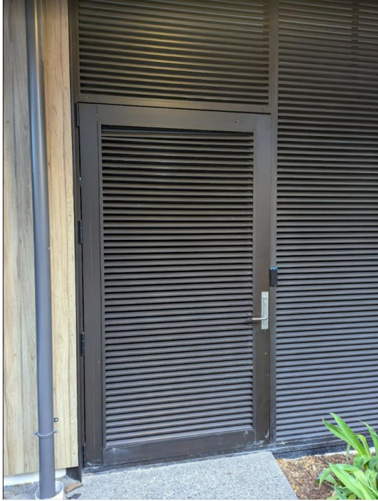
Cycle parking room 1: Access is via RFID reader, with residents offered RFID fobs on moving in. If a theft were to happen, the electronic record would show which fob was used at what time to access the bathroom to assist with Police enquiries etc
