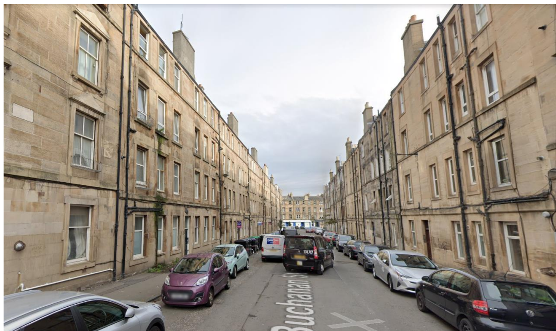
Above: Typical Georgian Tenements in Edinburgh (Google Street View)
