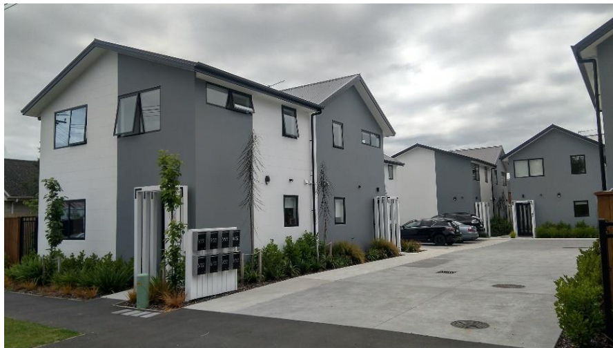
Figure 3: This development consisted of several smaller buildings (duplexes)
