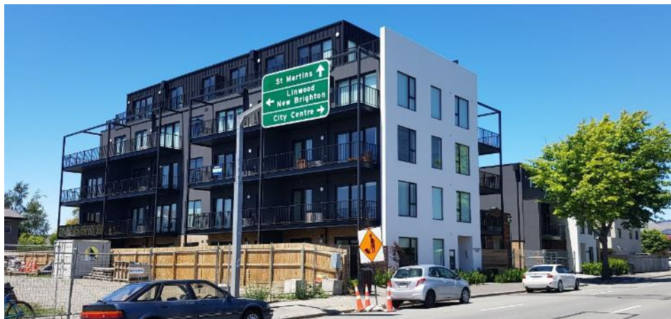
This building demonstrates visual interest and good materiality (but does overlook neighbours)
