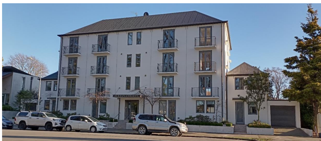
This building has a flat façade but vertical stacking of features clearly articulates the frontage.
