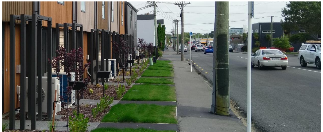
Above: Prominent HVAC units installed next to the street
