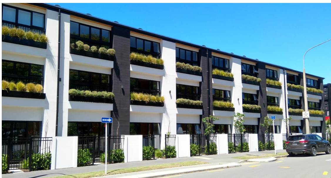
422 Hagley Avenue has enclosed balconies.
