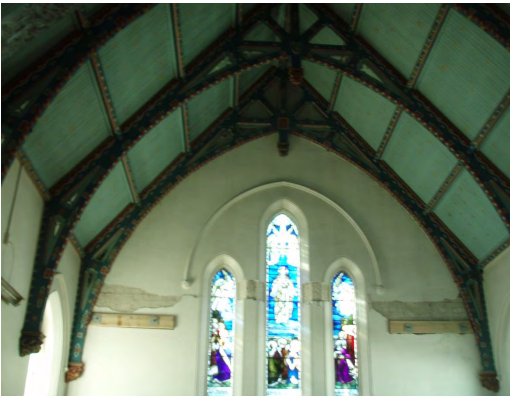
Photo 2a – Interior view of east gable – note cracking at nave wall eave level
