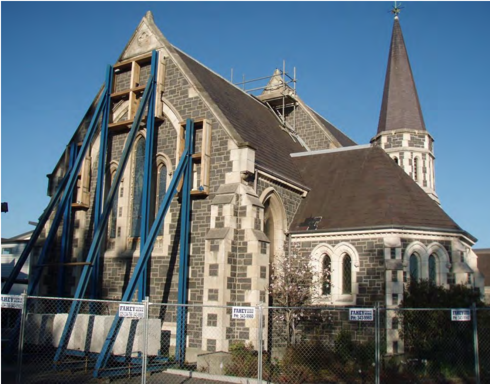
Photo 2 – Exterior view of east gable showing propping (west gable is similar)
