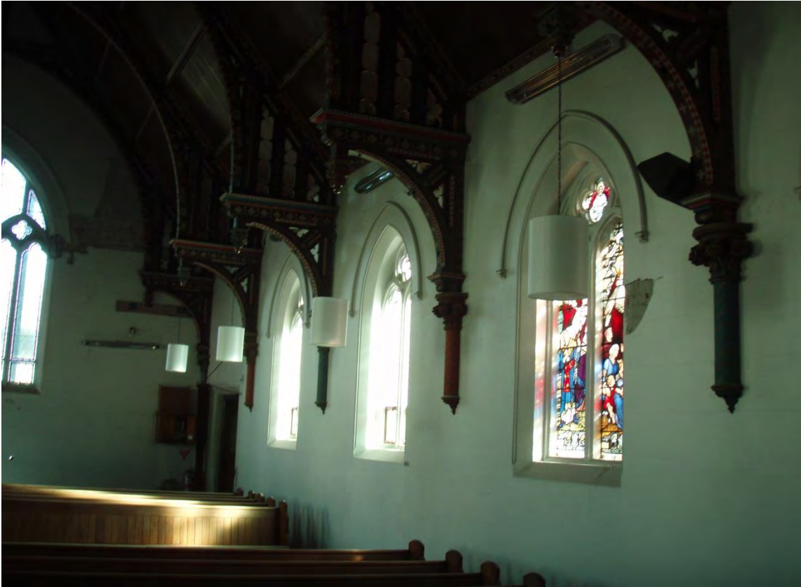
Photo 3 – general view of nave side walls
