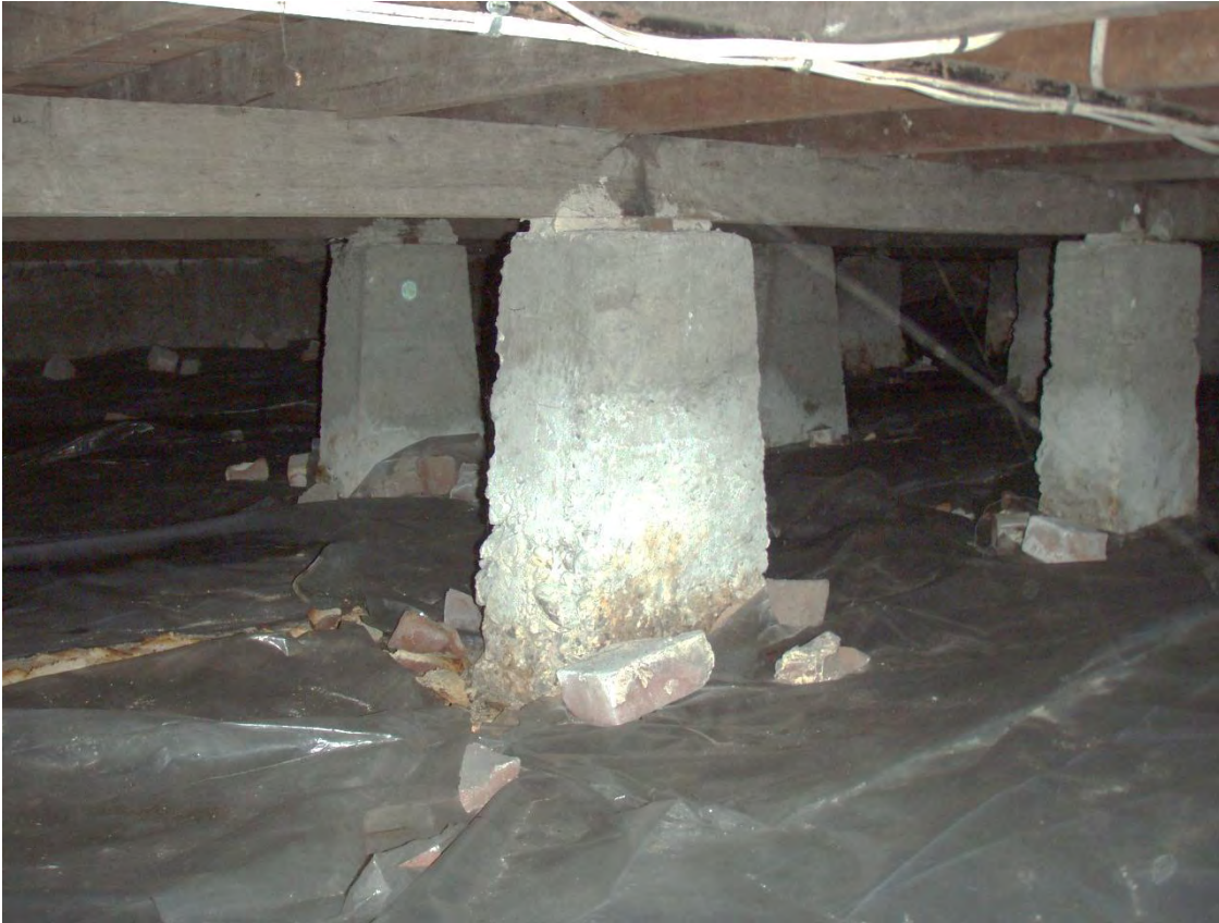
Photo 6 – General view under floor
