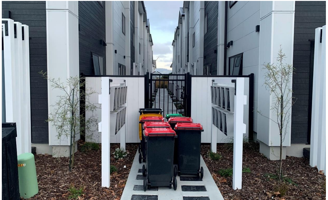
Figure 14 - 200 Worcester Street (Christchurch), 4.0m (approx.) total narrowest width - 1.5m path, 2 x 1.0 bin enclosures, and 2 x .25m garden edges.
