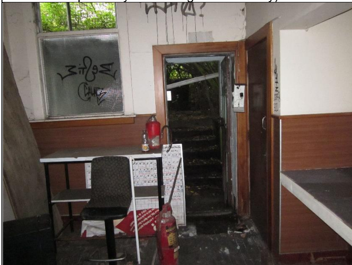
Photo 11 – View from interior. Another access to rear part of the building. It would appear the building had been assessed by others.
