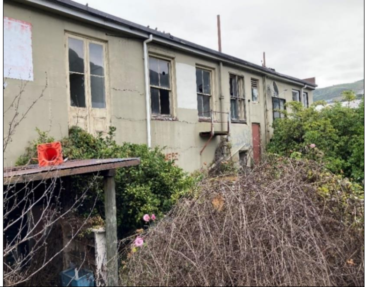
Photo 4 –View from Rear (North)
