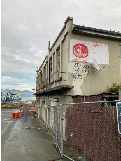
Photo 3 – View from East side wall
