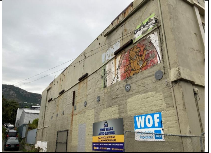
Photo 2 – View from West side wall
