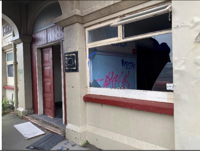
Photo 1 –View from the front (South)
