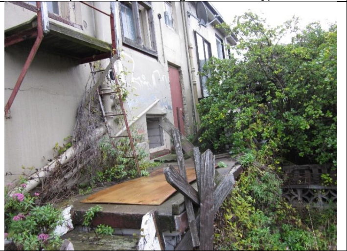
Photo 10 - Access to the rear part of the building
