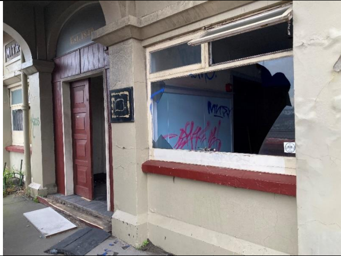
Photo 1 –View from the front (South)
