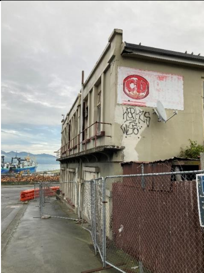
Photo 3 – View from East side wall
