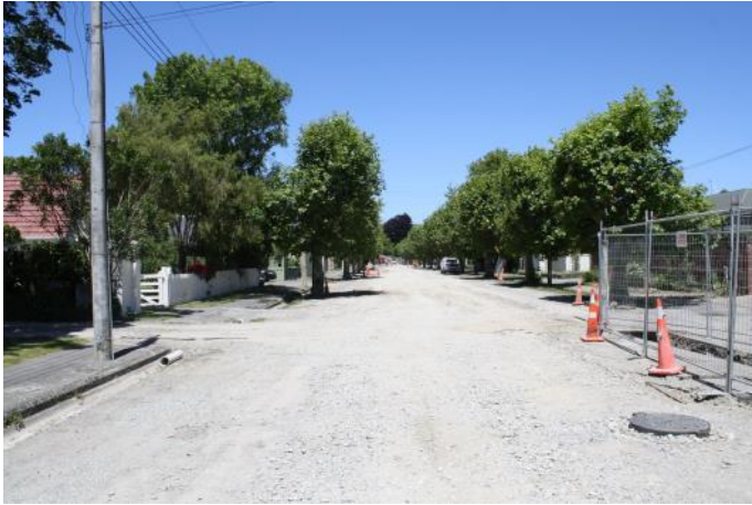
Garden Road Streetscape
