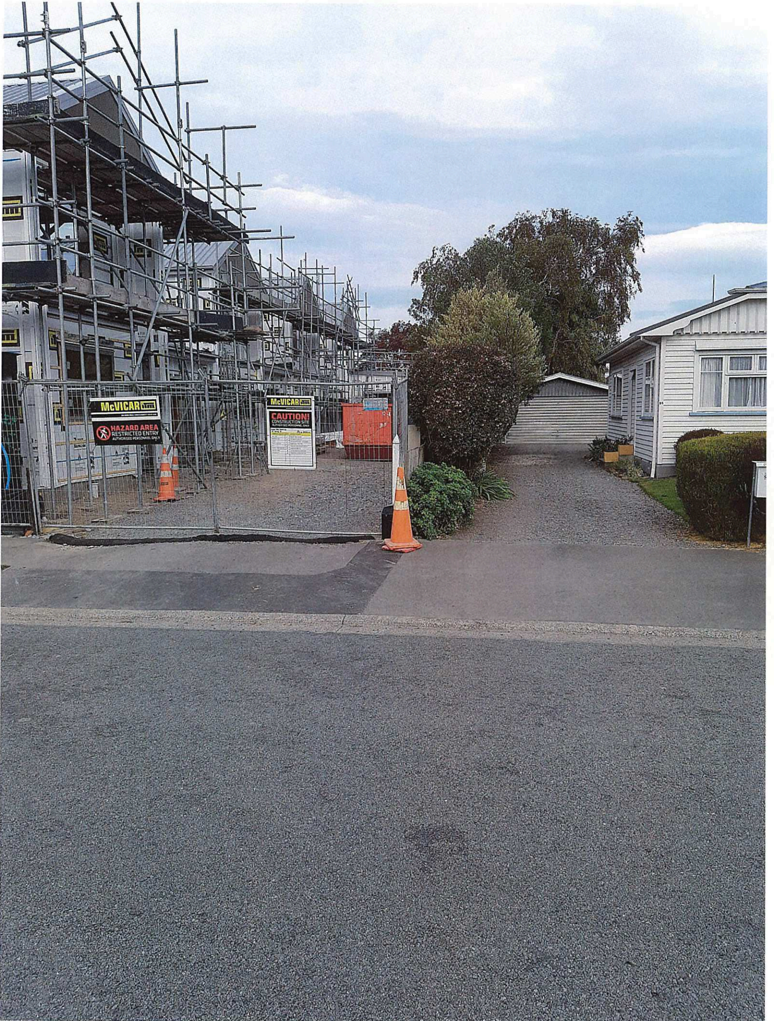
20 Haver Street - West side
