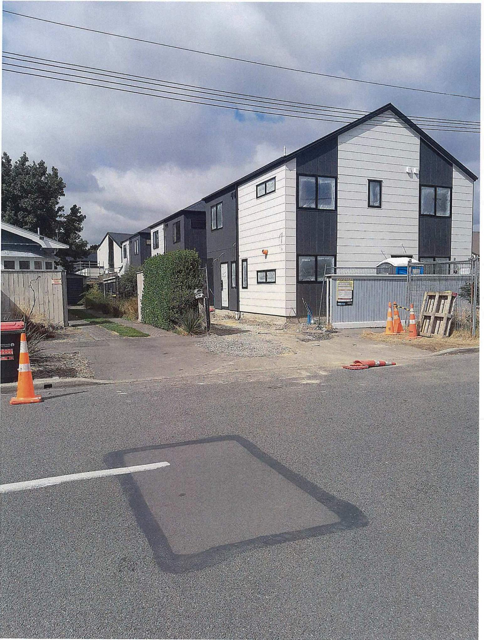
(4 apps) East side of 60 Frank St construction
