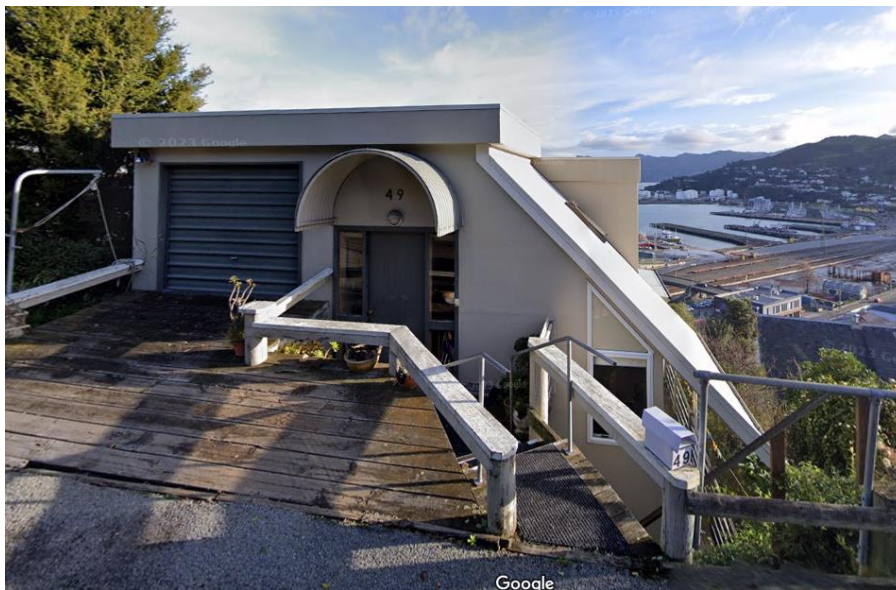
Figure 4: Existing street elevation (Source Google Streetview)
