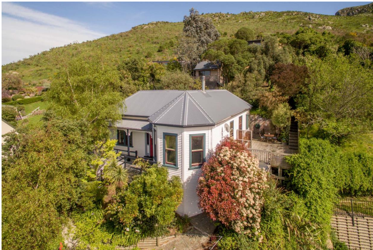
Figure 1: Existing residential unit
